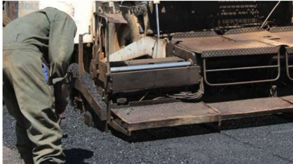
Road construction in Nakuru. FILE PHOTO | NMG
